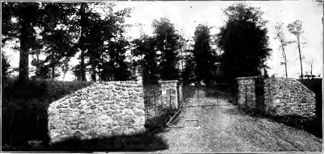
FIG. 250—STONE ANCHOR-WALLS FOR FENCE.
